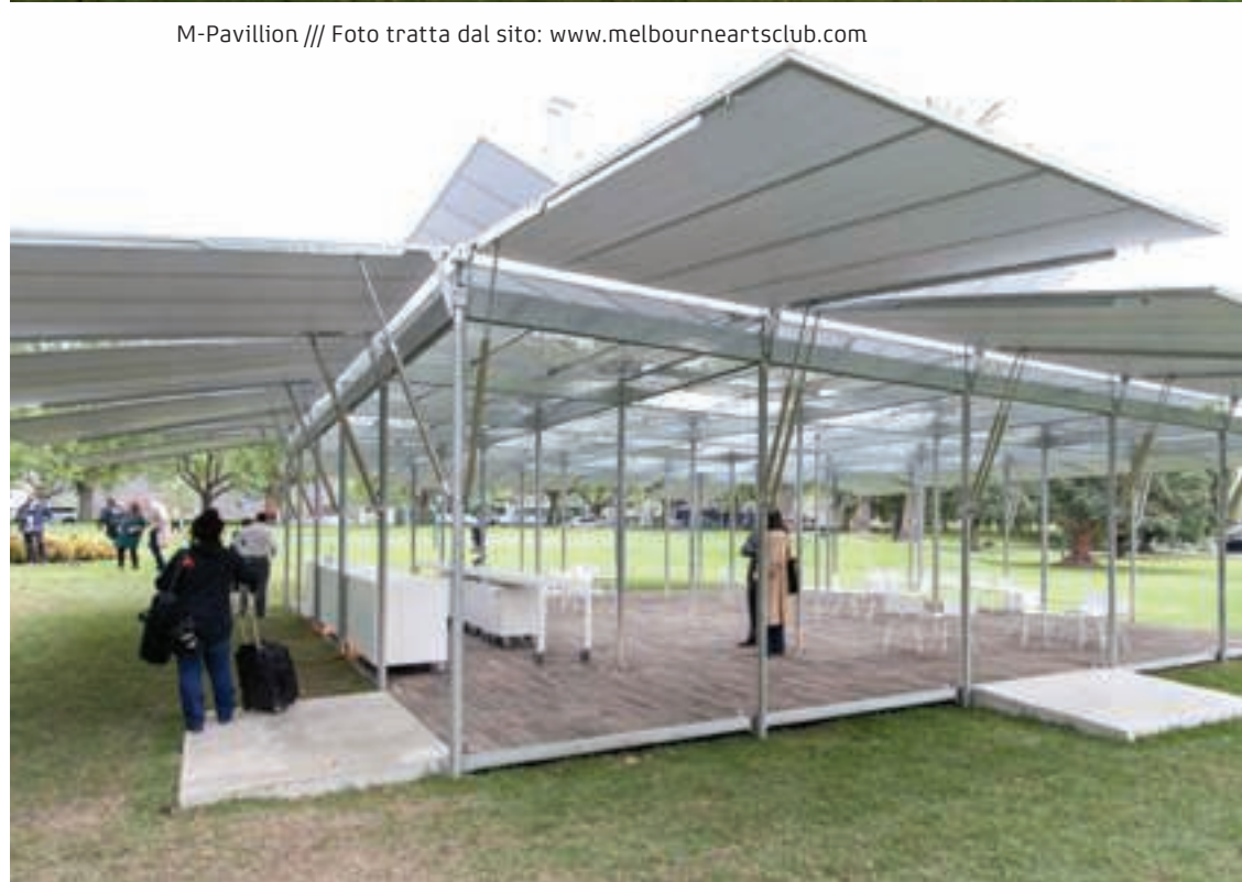
M-Pavillion /// Foto tratta dal sito: www.archdaily.com photo credit Earl Carter, courtesy of Sean Godsell Architects.
