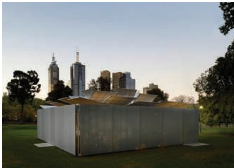
M-Pavillion /// Foto tratta dal sito: www.archdaily.com photo credit Earl Carter, courtesy of Sean Godsell Architects.
